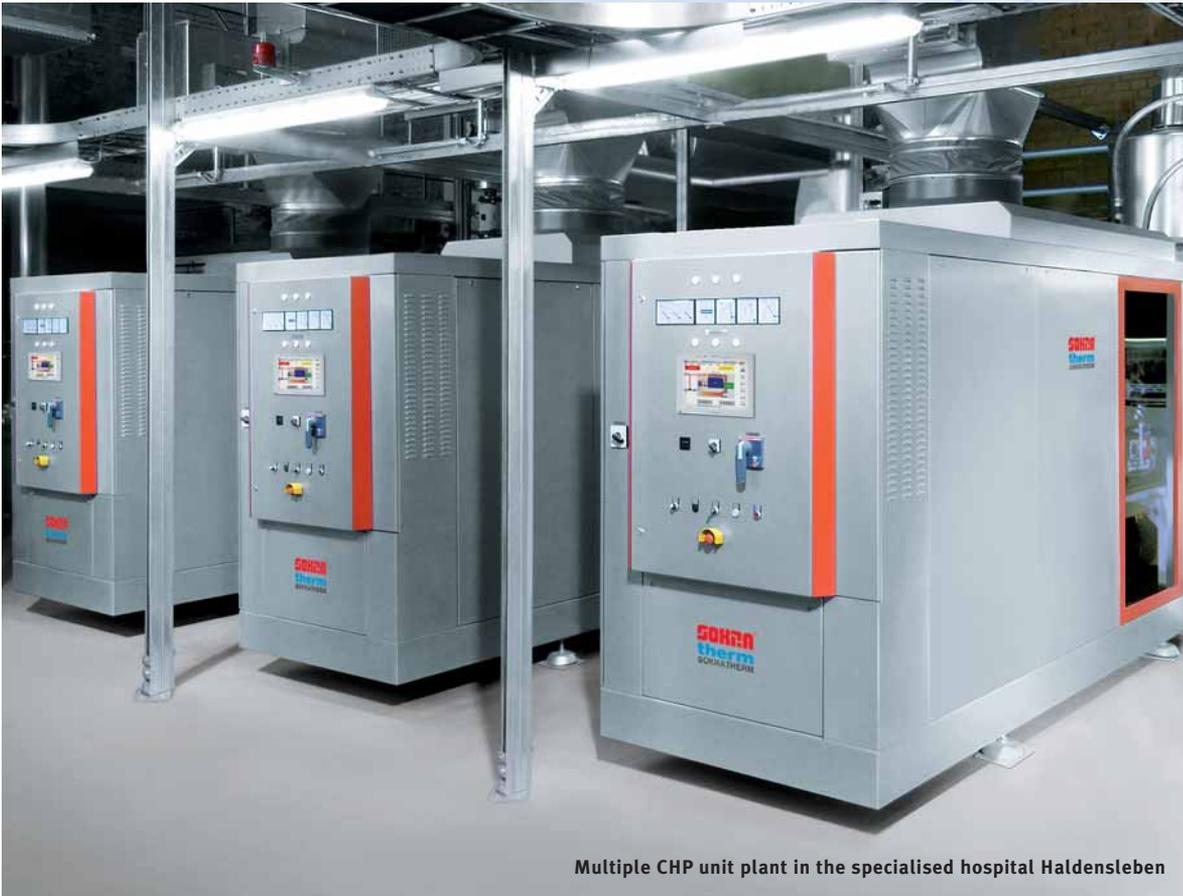
The combination of multiple CHP units allows an energy supply in the power range of Megawatts.
